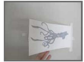
5) Rip the opposite tape tab leaving one half on the wall and the other on the graphic for re-alignment purposes.
